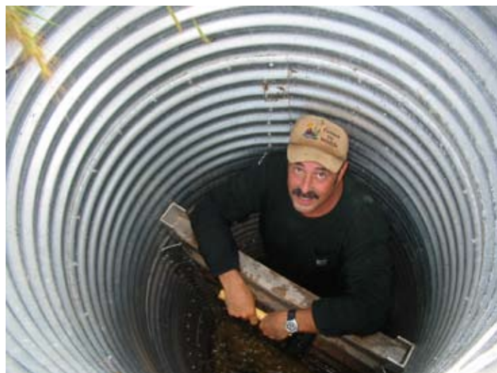
Jeff Nania of Wisconsin Waterfowl Association inserts stop boards at the 4 acre wetland north of Kampen Rd.
